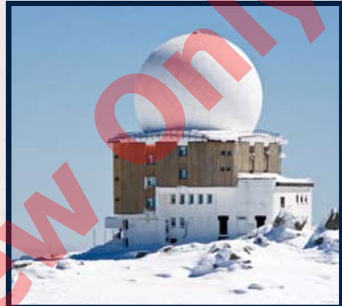
A radar in the dome on top of this weather station uses radio waves to track precipitation.
